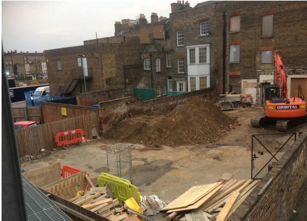
Image 1.2 - Existing Site Image (looking southwest – Source: LPA Case Officer)
